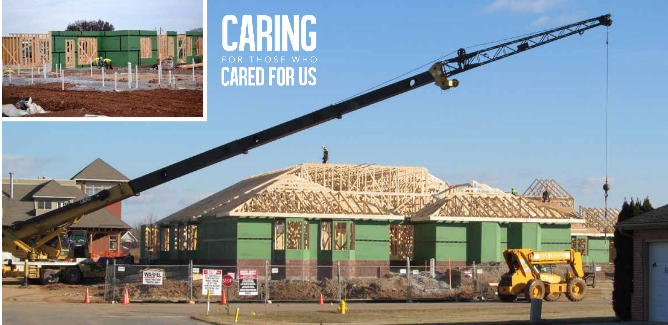
MAIN: Capital Campaign donations at work as construction begins on SpiriTrust Lutheran™, The Village at Sprenkle Drive expansion project. TOP LEFT: Construction employees spread concrete at the site of the new Assisted Living residence at SpiriTrust Lutheran, The Village at Sprenkle Drive.
